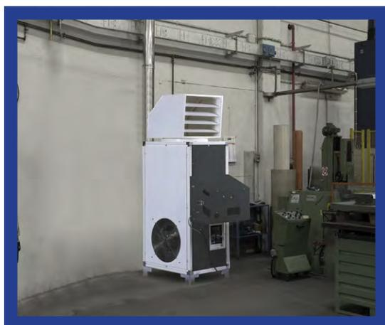
*Burner is supplied with snorkel outlet to ensure clean combustion air through connection with external air aspiration duct*
